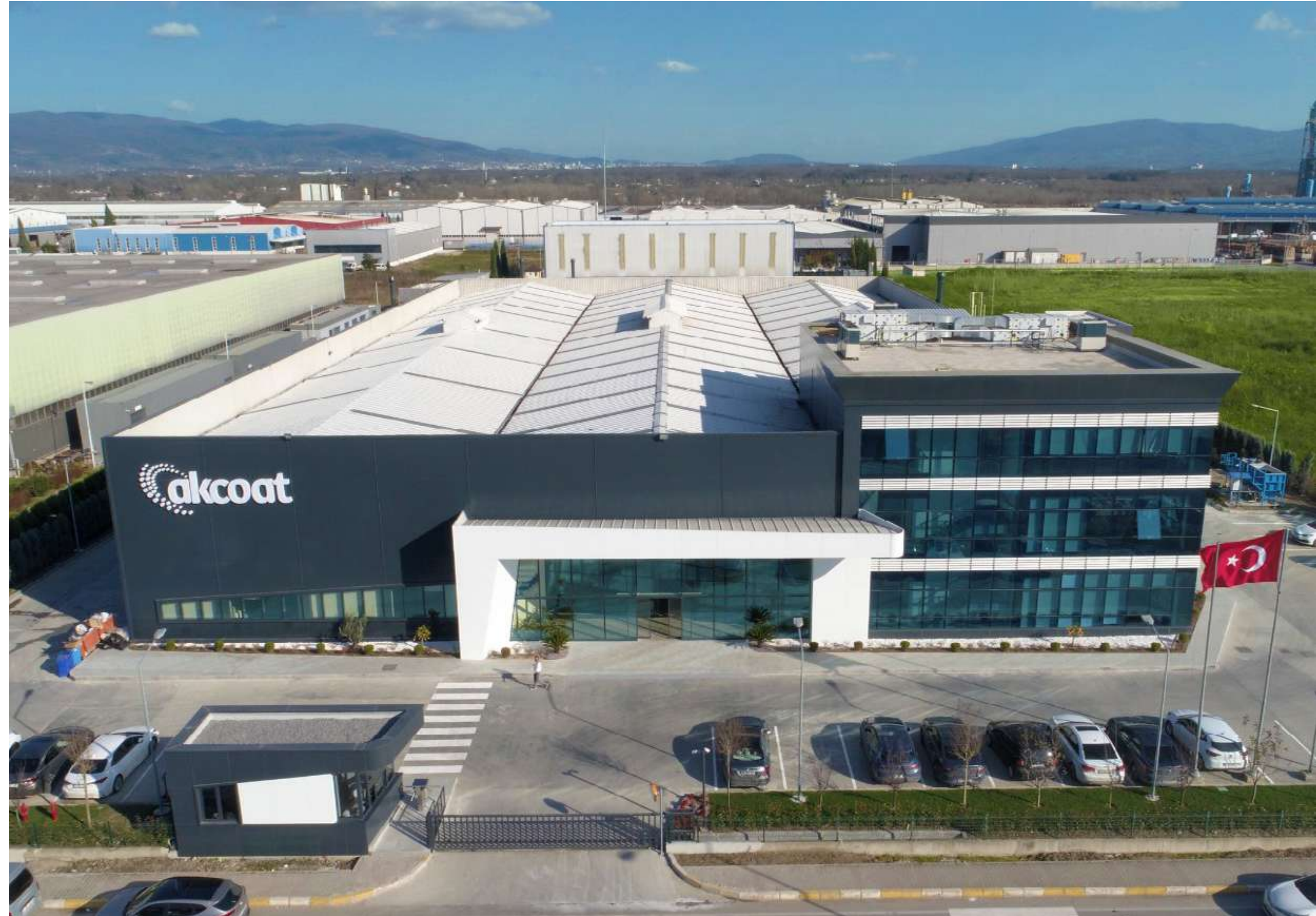
Akcoat Facility, Sakarya
