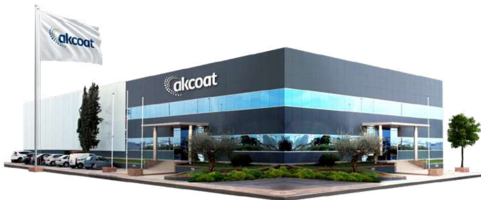
Akcoat Facility, Spain
